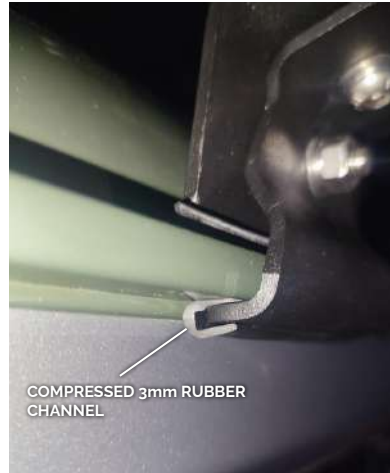
Figure 7: Completing gutter mount fitment
